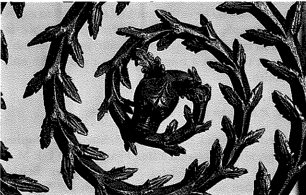
This intricate spiral of iron was wrought from one piece of metal, with no welding.
